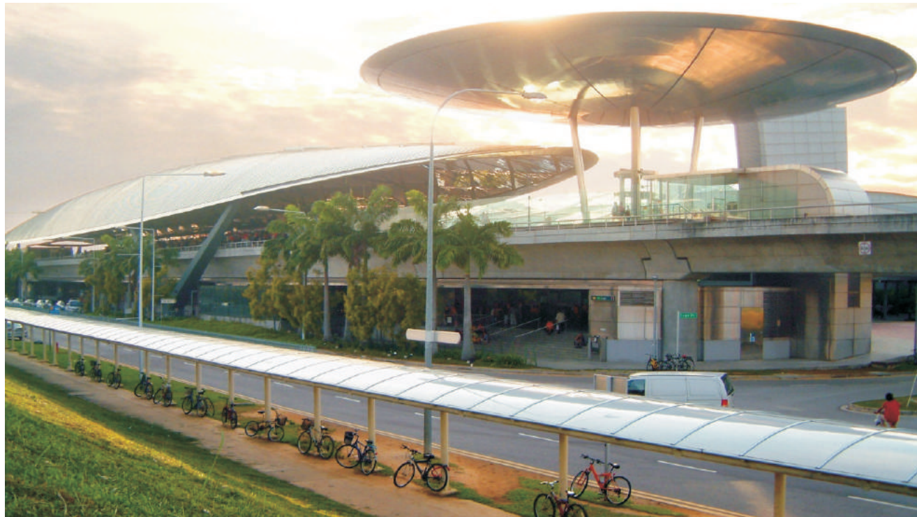
LTA Metro Station
