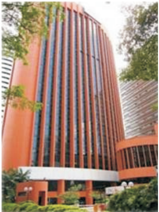
Malaysia Menare ING 22nd Floor / Station 4.0m/s
