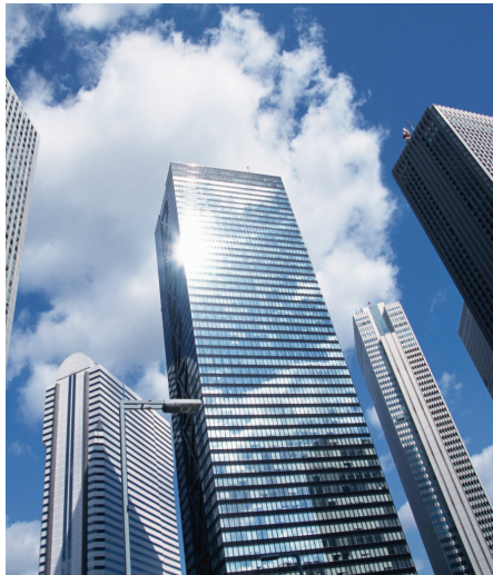
Guofeng Building, Taiyuan Guofeng Building 27 floors/station 3.0m/s
